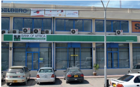
Airport Branch, in Dar es Salaam.
